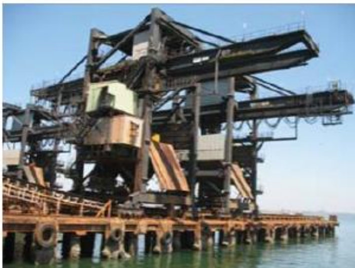
Figure 32. Tyres abutting jetty when filled with rain water can be extremely dangerous in providing the first foothold to any mosquito arriving with a ship © Ashwani Kumar
